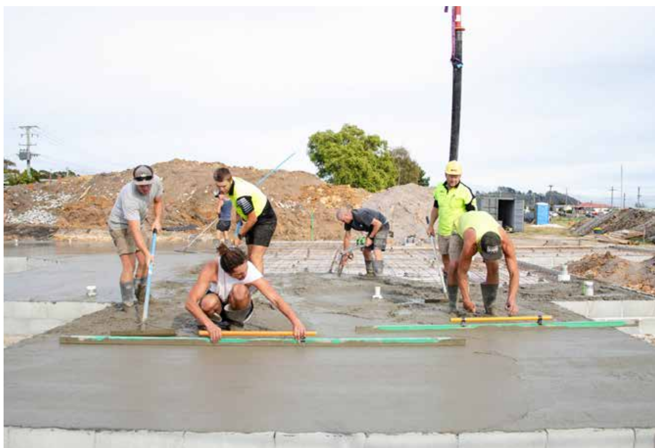
2B Build laying the slabs for the Somerset properties
