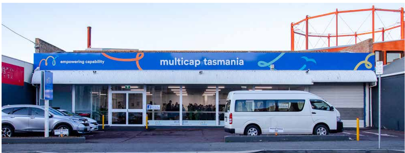
Launceston hub at 31 Tamar Street
