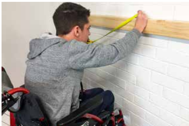
Luke thoroughly enjoyed buying the materials and putting up the foundations of the sensory wall
