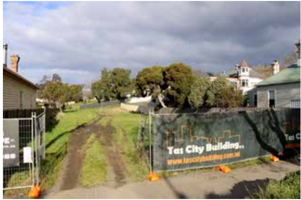
The site for the new homes in Dowling Street
