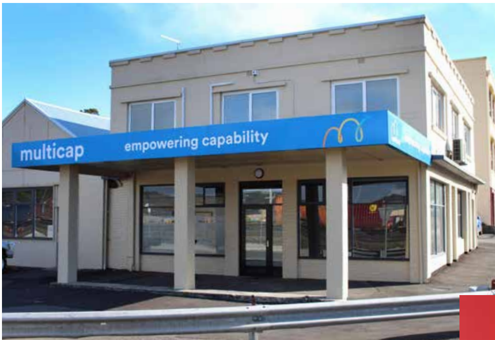
Multicap Tasmania's Burnie office at 35 Marine Terrace
