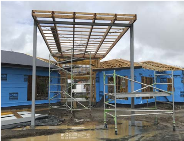
New group home being built in Pamela Court.
